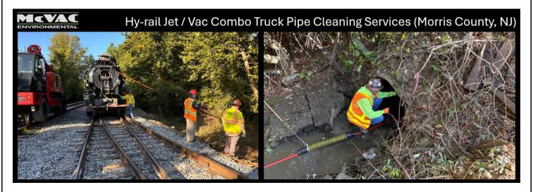
On this project, McVAC utilized the Hy-rail Jet / Vac Combo Truck to clean existing 36" to 48" reinforced concrete pipe runs along / beneath the railroad tracks as directed by the General Contractor. Water was decanted from the debris body, and subsequently the solids were transported off-site for disposal.
